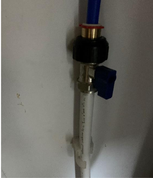
Picture above of what a valve looks like once connected to a coffee machine pipe.
